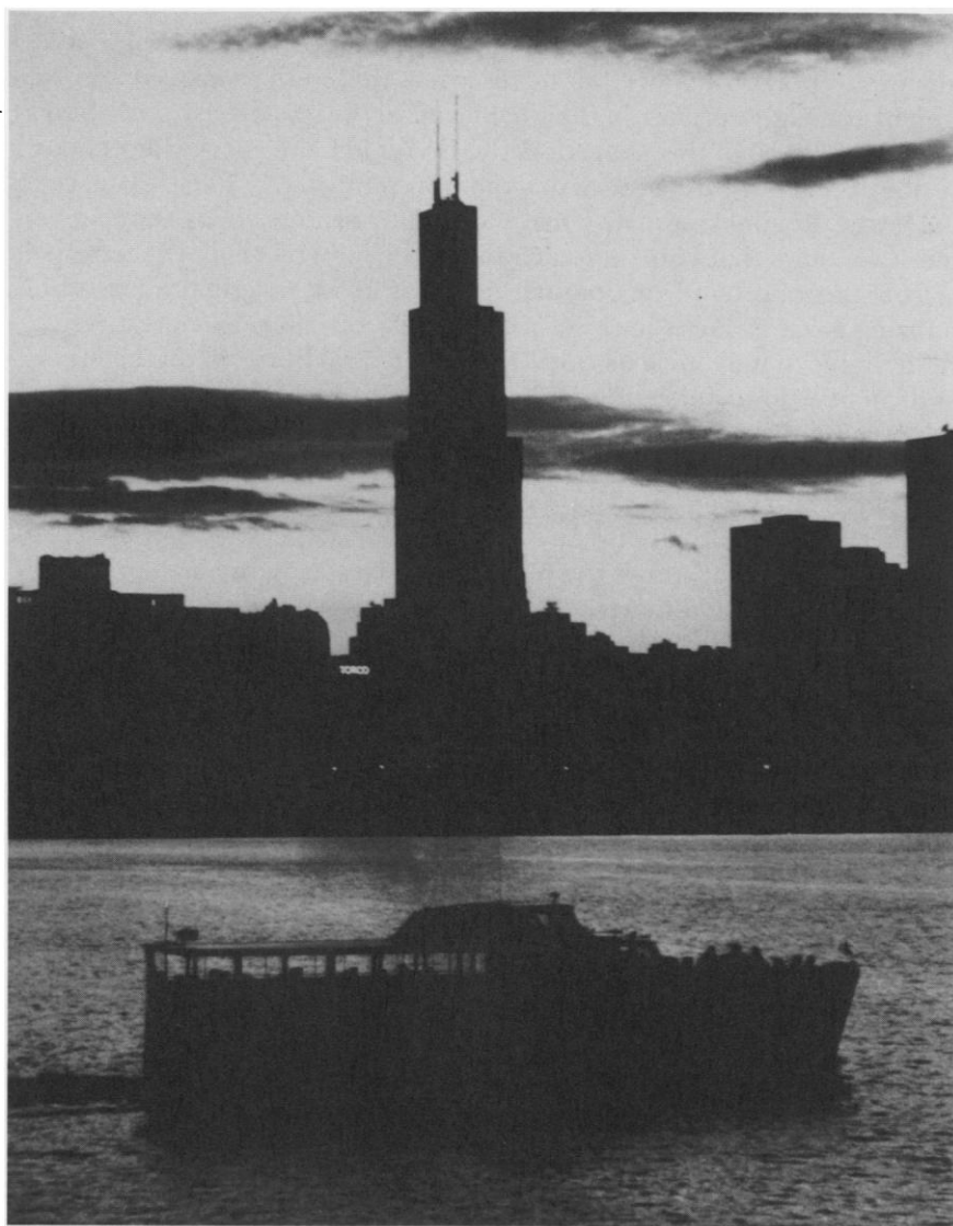
FIG. 2.—Photo: Illinois Distribution Company (CH-1189E).
